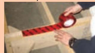
1 Installation on bond-breaking tape
