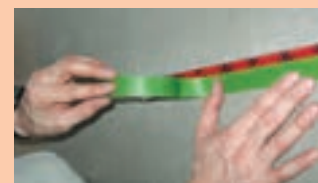
6 Installation of masking tape
