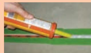
7 Application of flexible adhesive sealant
